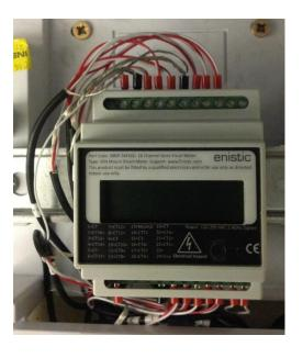
Note that connections 1,5,9,15 and 19 have the screening wire of multiple clamps connected to them
